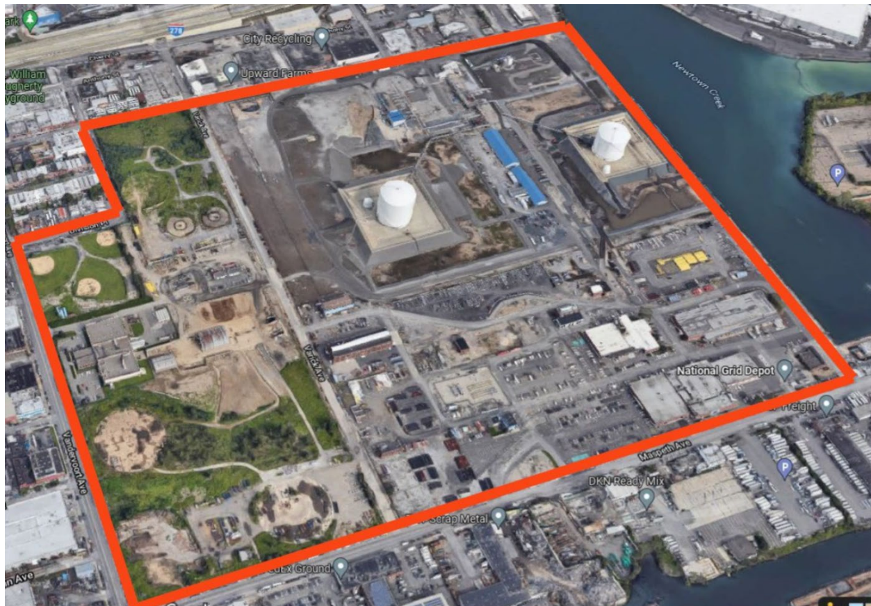
Figure 6-1: Greenpoint Energy Center
