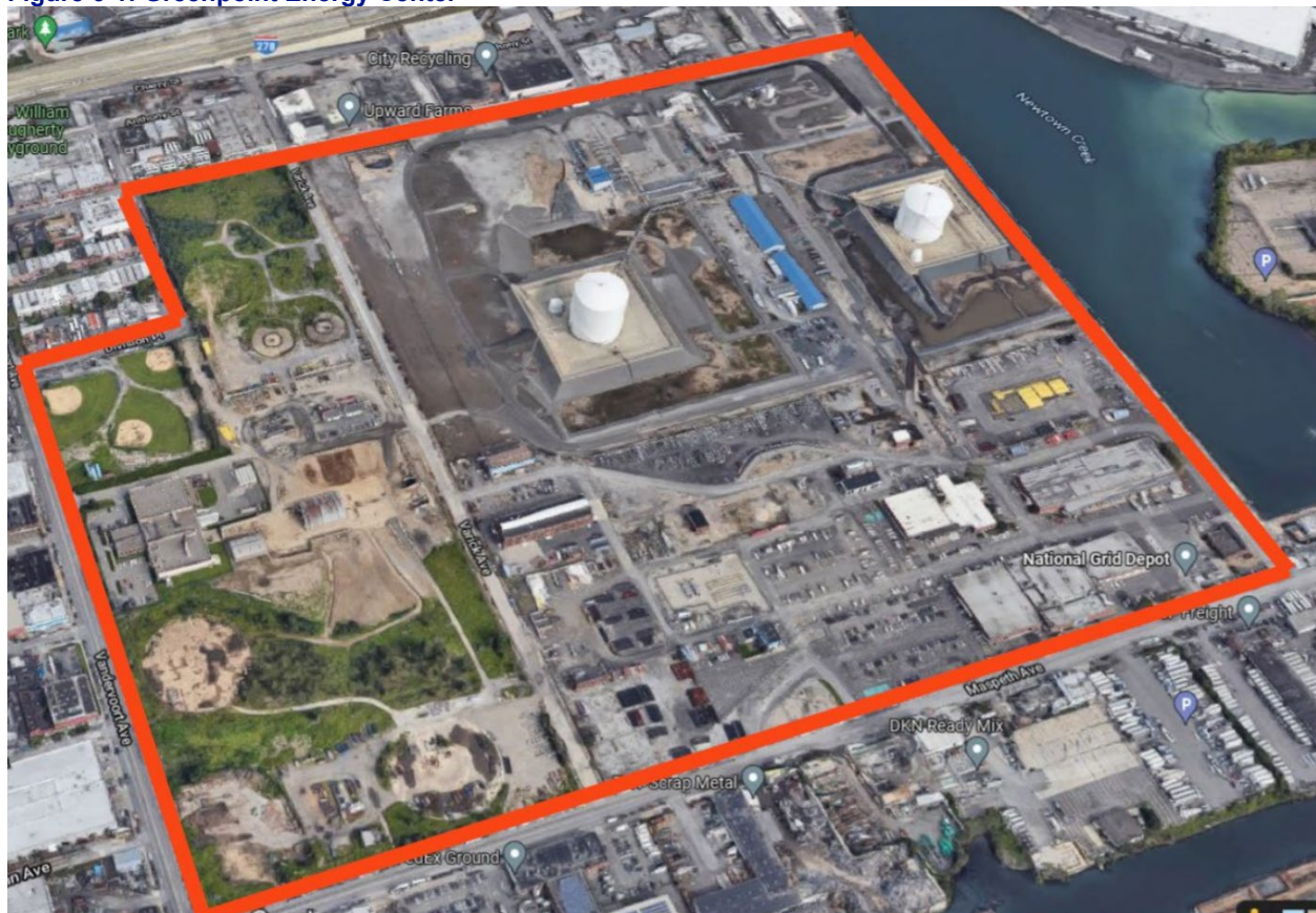
Figure 6-1: Greenpoint Energy Center
